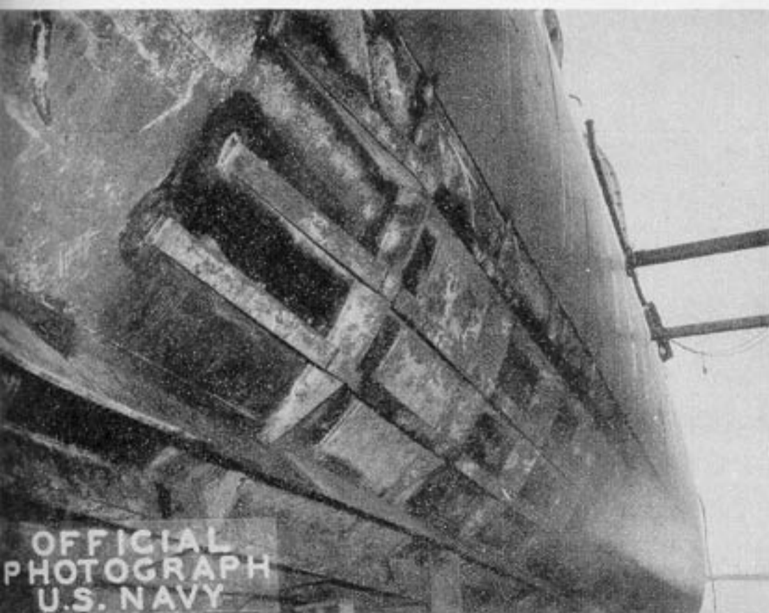
Photo 12-10 HUGH W. HADLEY (DD774). Port side looking aft following repairs in ARD28.
