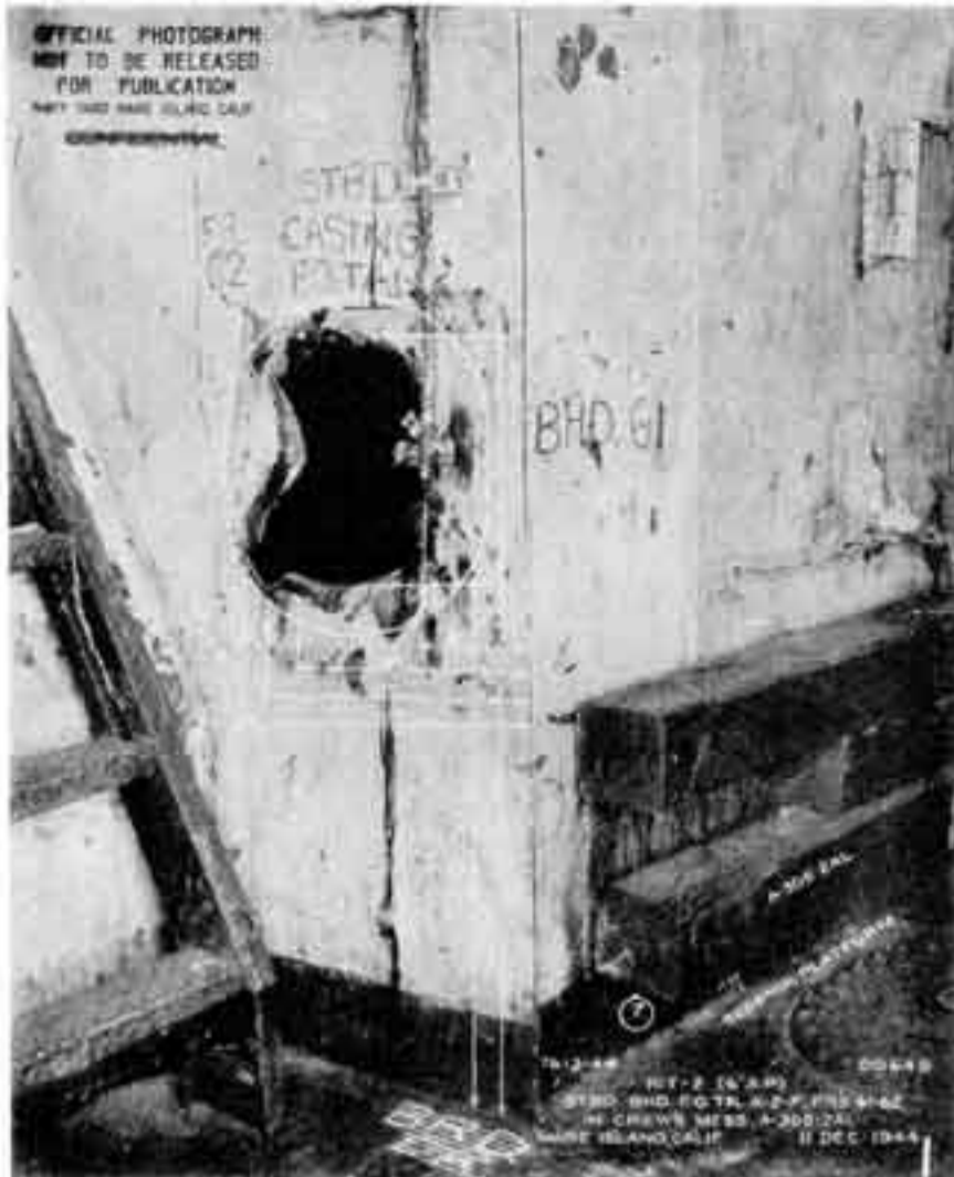
Photo 5-3: A.W. GRANT (DD649) - Hit #2. View looking aft at hole in forward starboard corner of A-2-F caused by 6-inch AP dud which passed through A-305-2AL. Shown looking aft on second platform.
