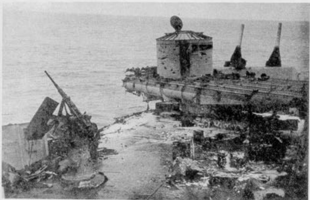
Photo 12-3: HUGH W. HADLEY (DD774). After torpedo mount, frame 163, showing fragment damage. Foam used in fighting fire is in foreground.
